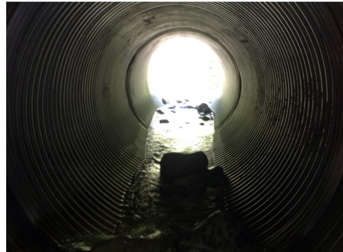
looking through culvert
